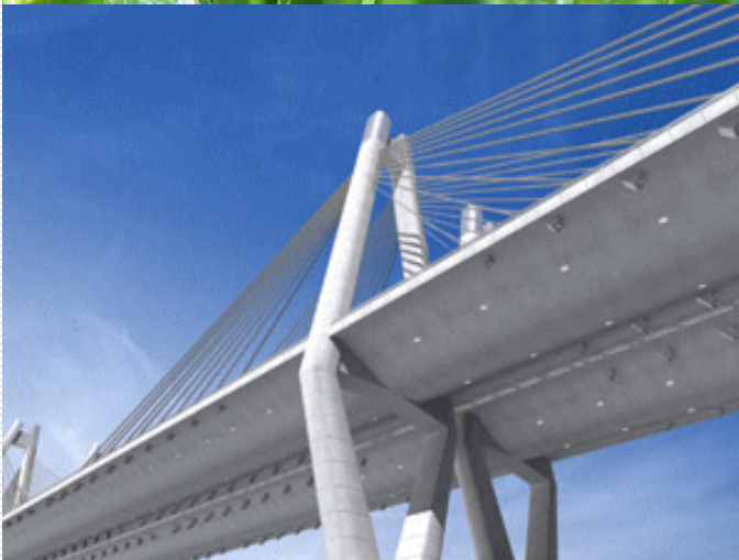
Bridge Mumbai, India
