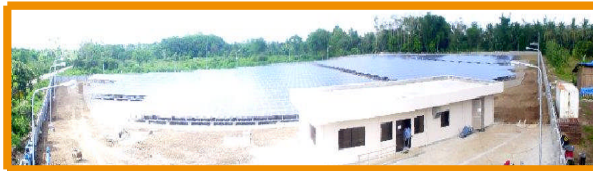
Stage 3: Completed plant; Commercial Operations – Sept. 2004
