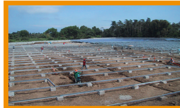
Stage 2: Panels being installed
