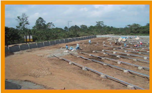
Stage 1: Initial site work
